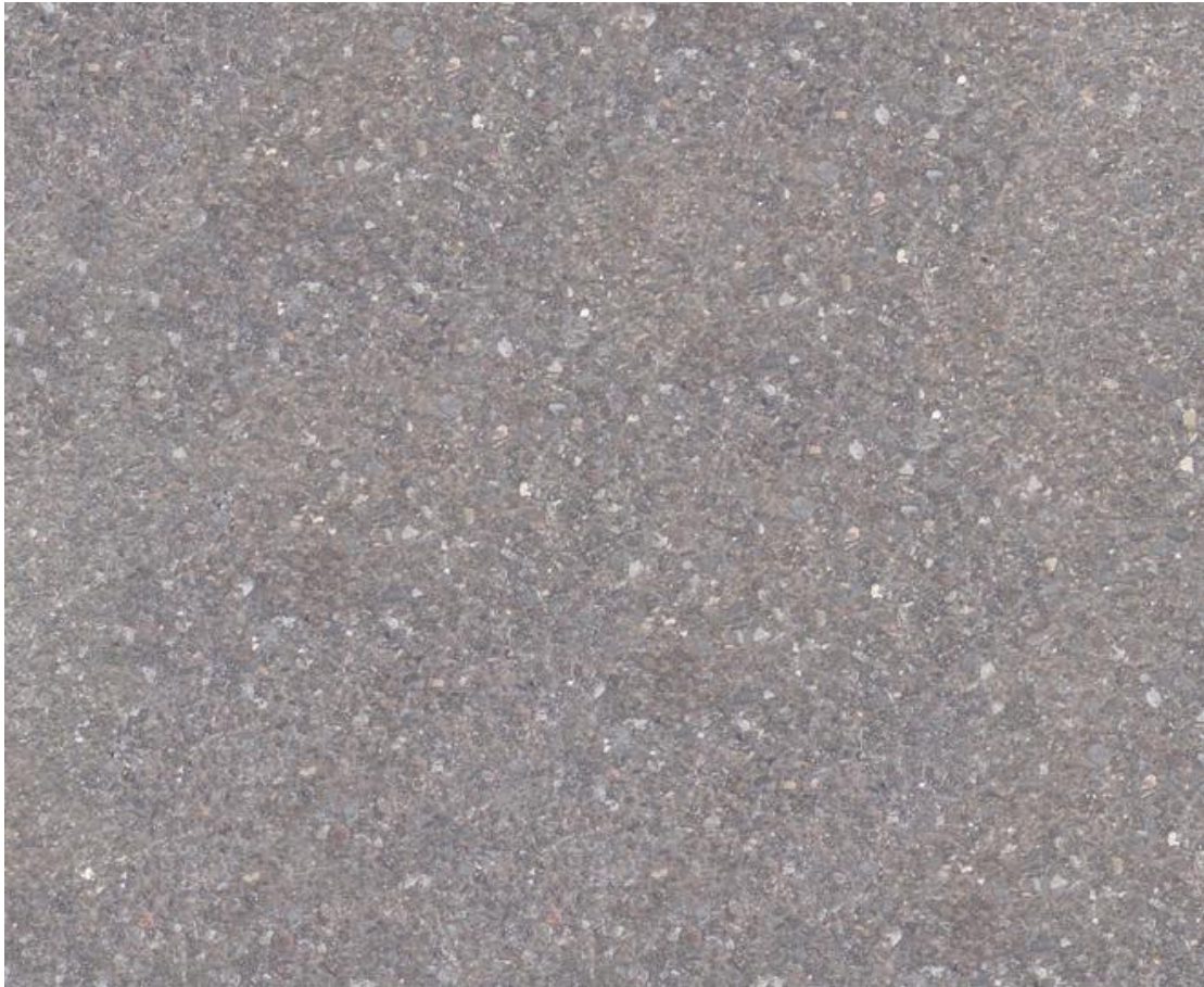
Dense Bitumenous Mix- Very Little Exposed to Weathering
